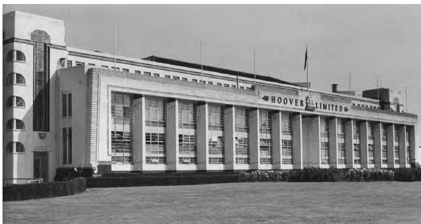
Plate 217 Former Hoover Factory by Wallis, Gilbert, & Partners, on Western Avenue, London, of 1931–32. The long front with battered sides is a version of an Egyptian temple-front, whilst loculi-like openings are recalled in the windows of the towers (which also sport a tall window with head composed of the chamfered or canted pseudo-arch). The Piranesian stepped motif also recurs in the centrepiece. Photograph of 1980 (JSC).
